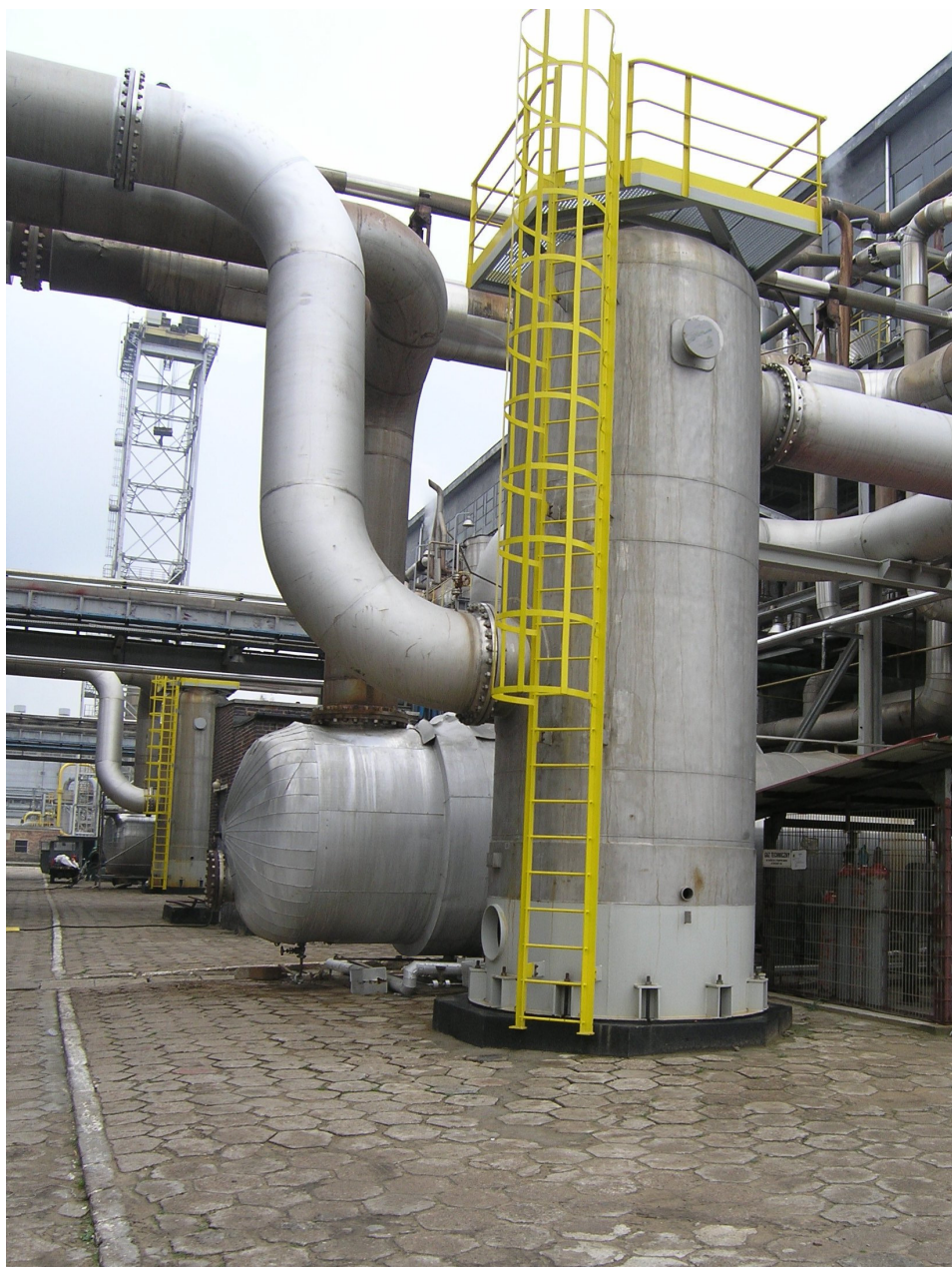
Fig. 5. Condensate separator from tail gases
